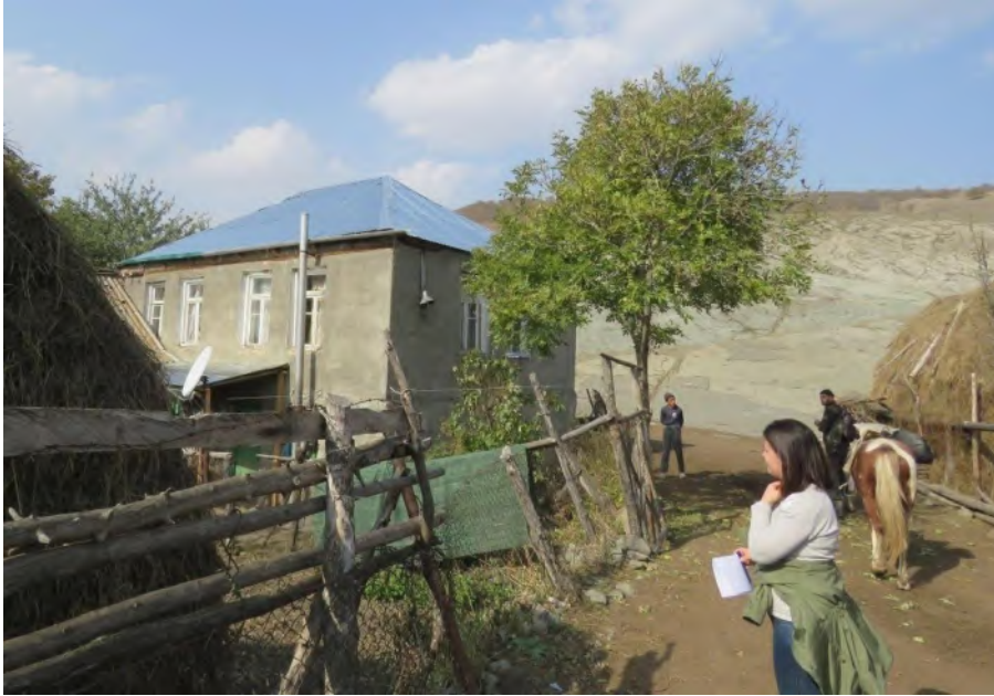
Figure 30. House with renovated roof in Napilnari village
